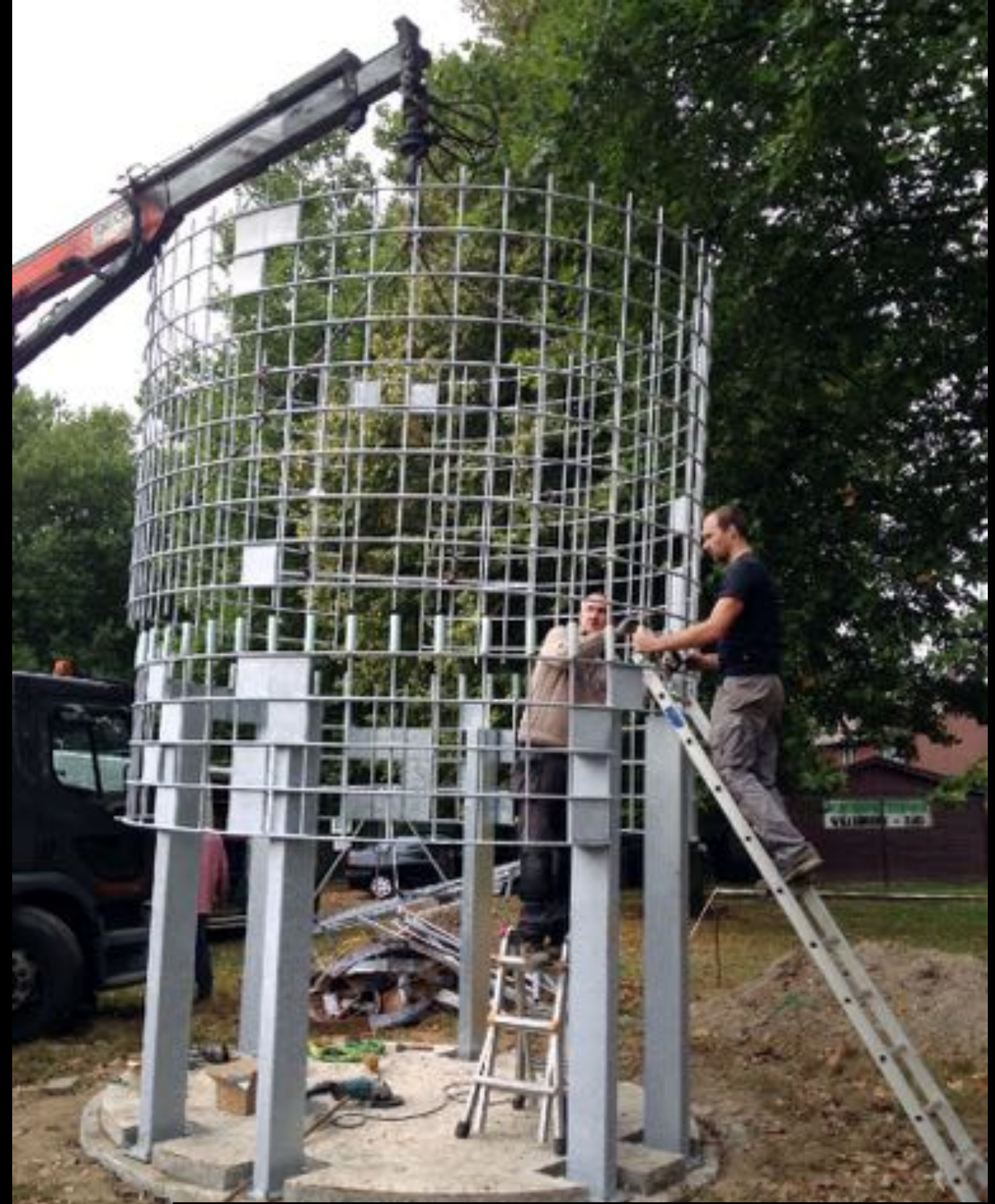
SEADS, Kris Mys & Compostmeesters Willebroek, Biodiversity Tower , 2015 Foundations and construction process
