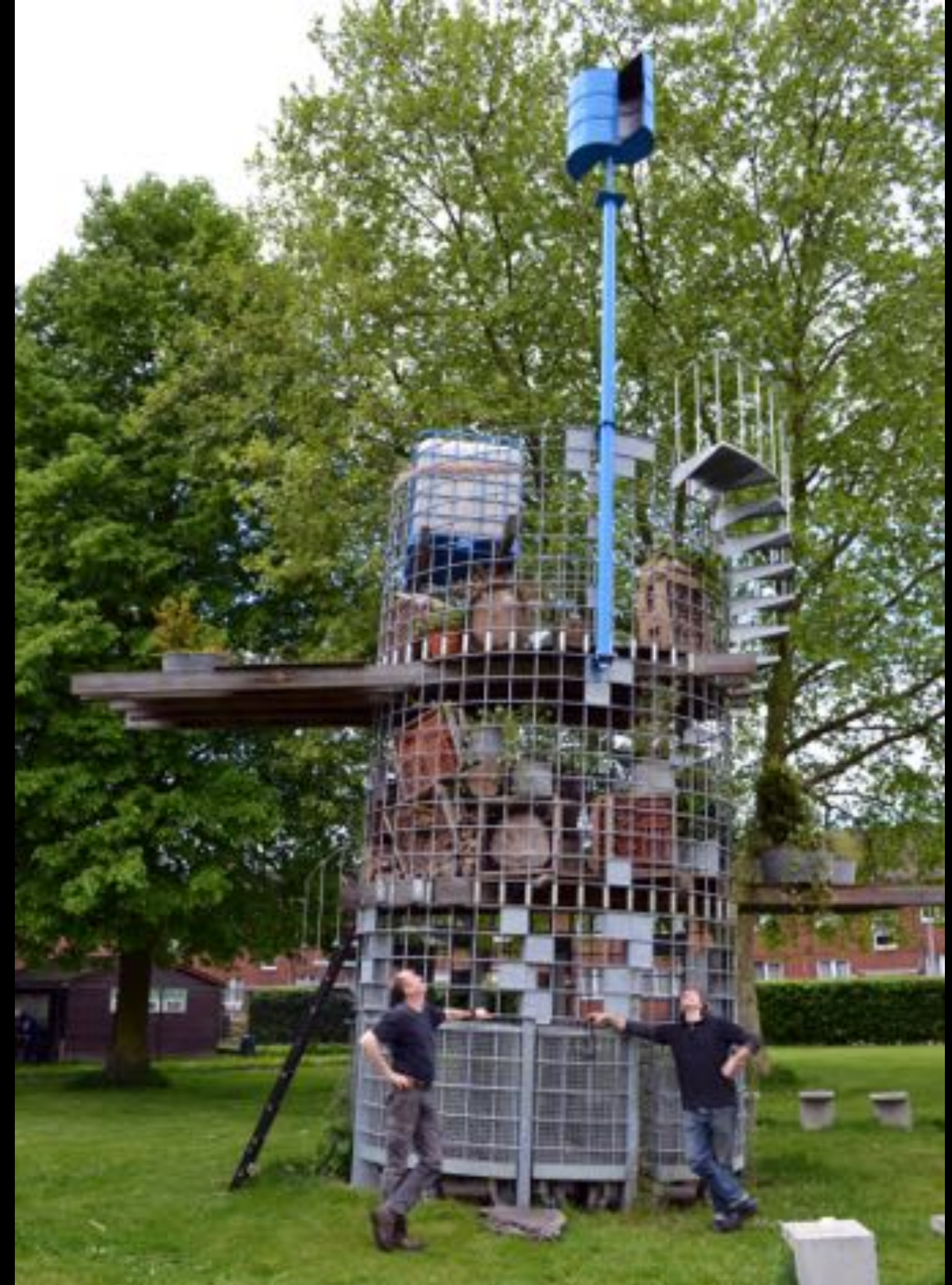
SEADS, Kris Mys & Compostmeesters Willebroek, Biodiversity Tower , 2015 Installment of Savonius wind turbine for the water pump
