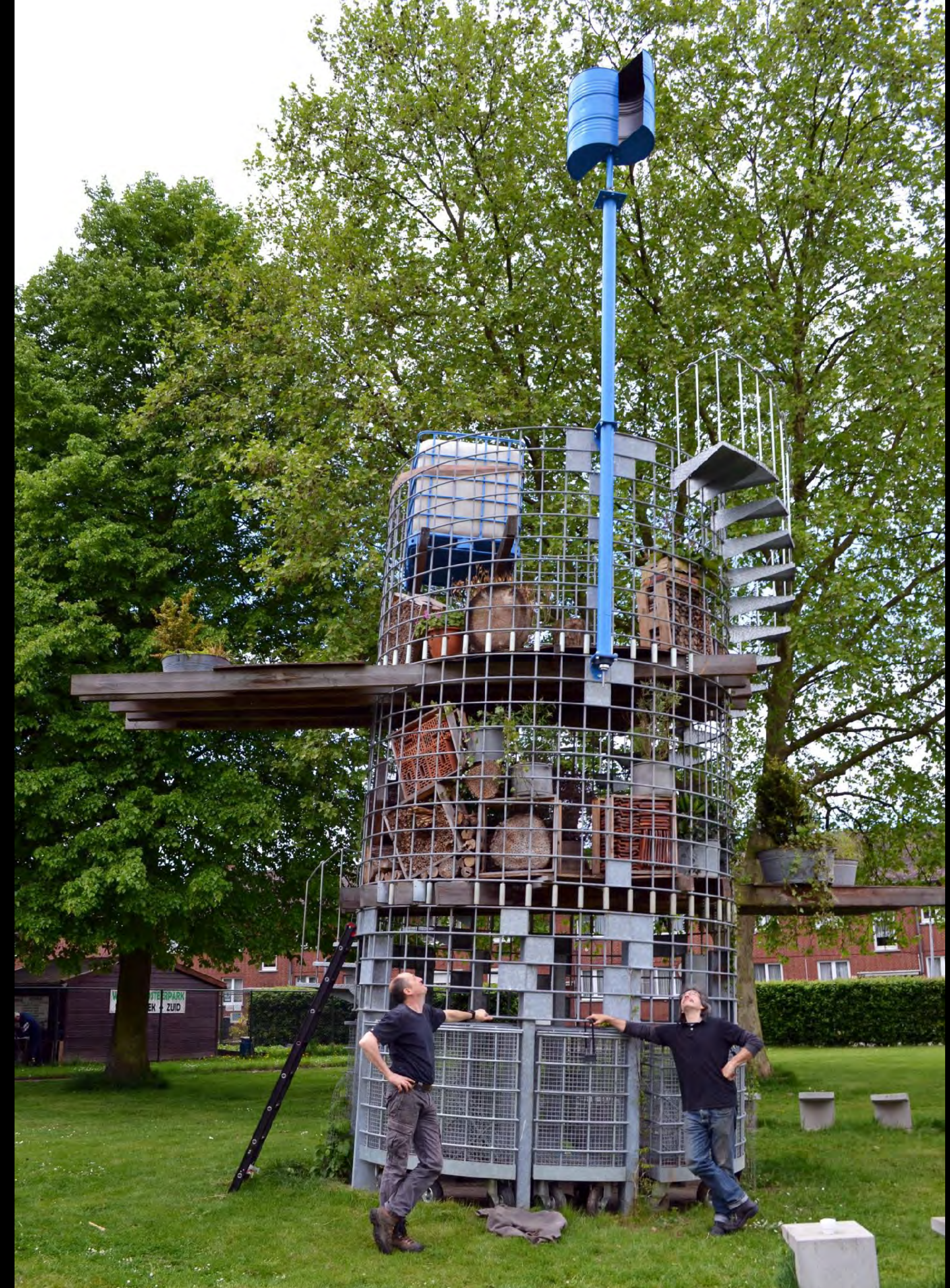
SEADS, Kris Mys & Compostmeesters Willebroek, Biodiversity Tower , 2015 Installment of Savonius wind turbine for the water pump
