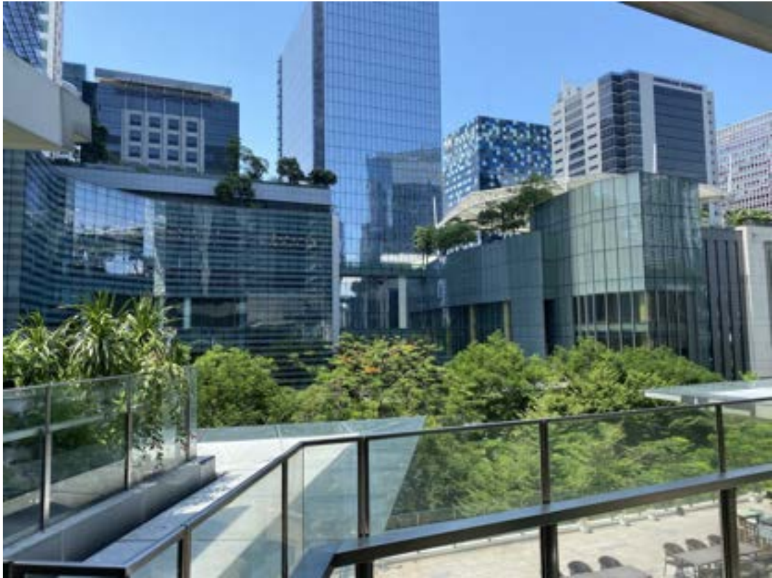
Figure 37: Green Roofs and Rooftop Gardens, BGC
